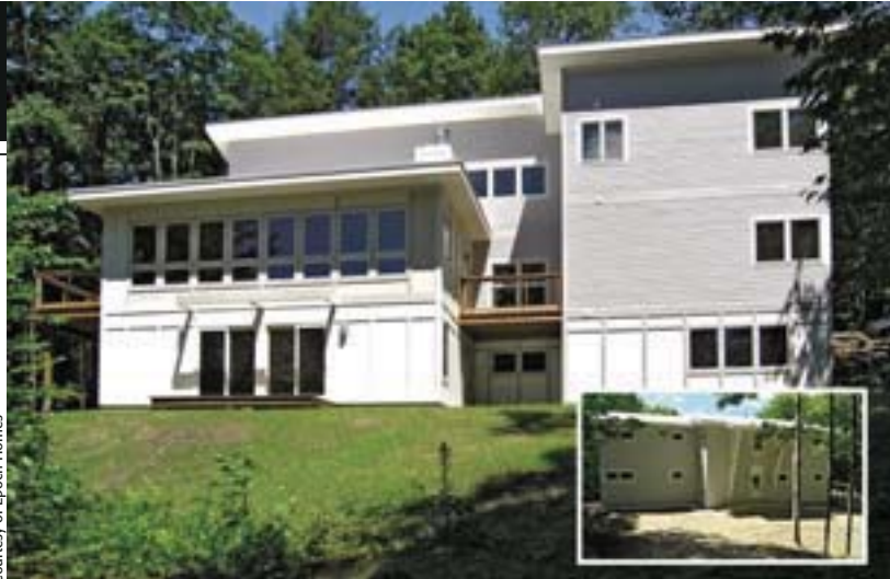
One of the Platinum LEED certified homes built by PowerHouse Enterprises and Epoch Homes.
